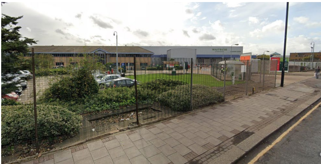
Figure 4: Existing poor streetscape along Southbury Road
